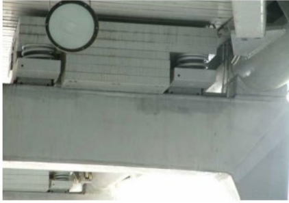
Tuned mass dampers beneath the bridge platform.
