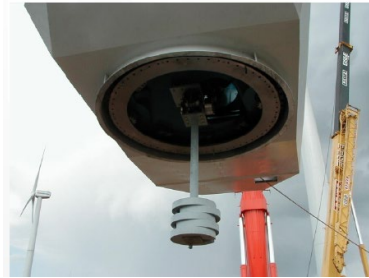
Tuned mass dampers beneath the bridge platform.
